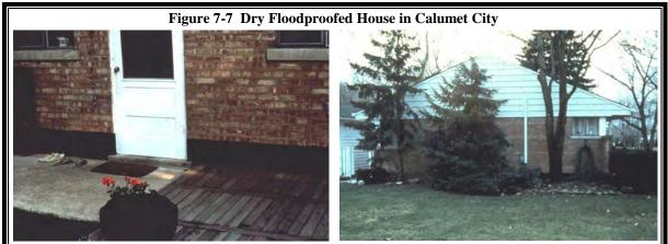
This project kept water out during the 1982 flood and proved that it was one of the most cost effective floodproofing projects ever made. While the waterproofing compound left a black strip over the lower rows of brick, it was hidden by planting and landscaping in the front and side yards.
