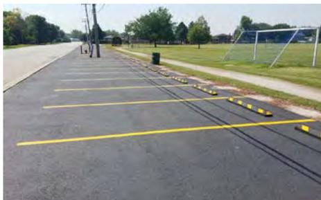
Sealcoating and striping, along with new stop blocks, at Paarlberg Park and sealcoating of Veterans Park maintenance driveway.
